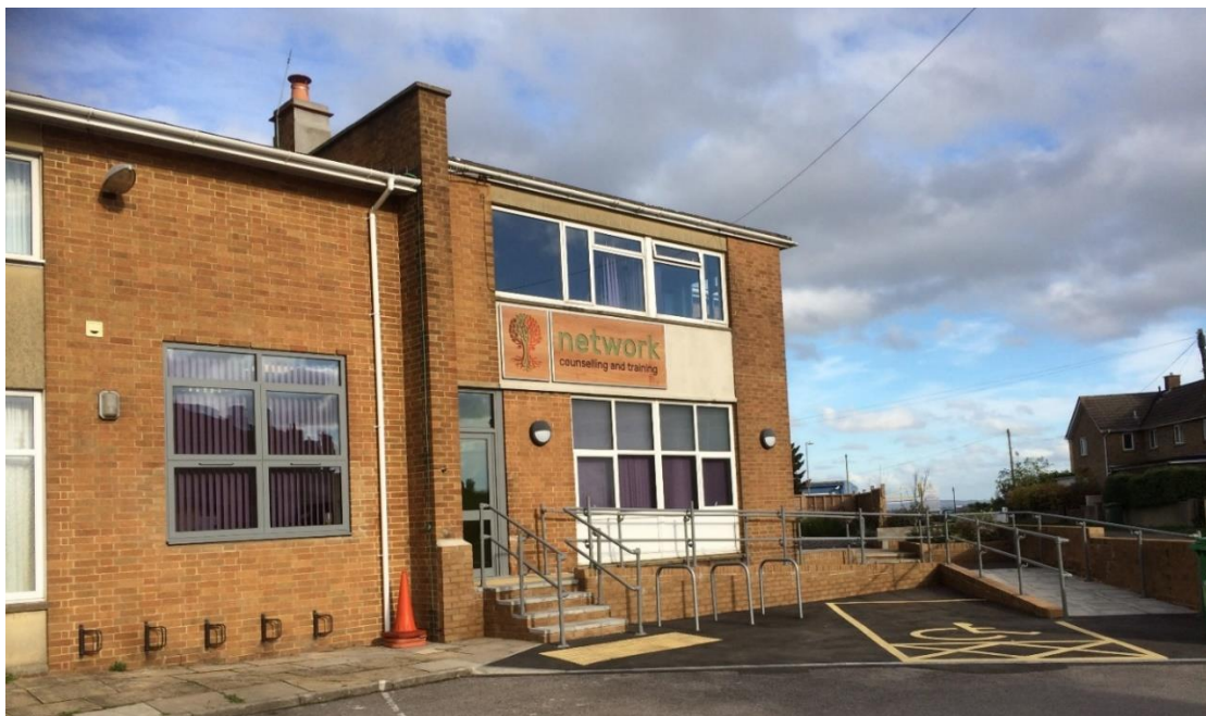
Network at Elm Park, Filton
