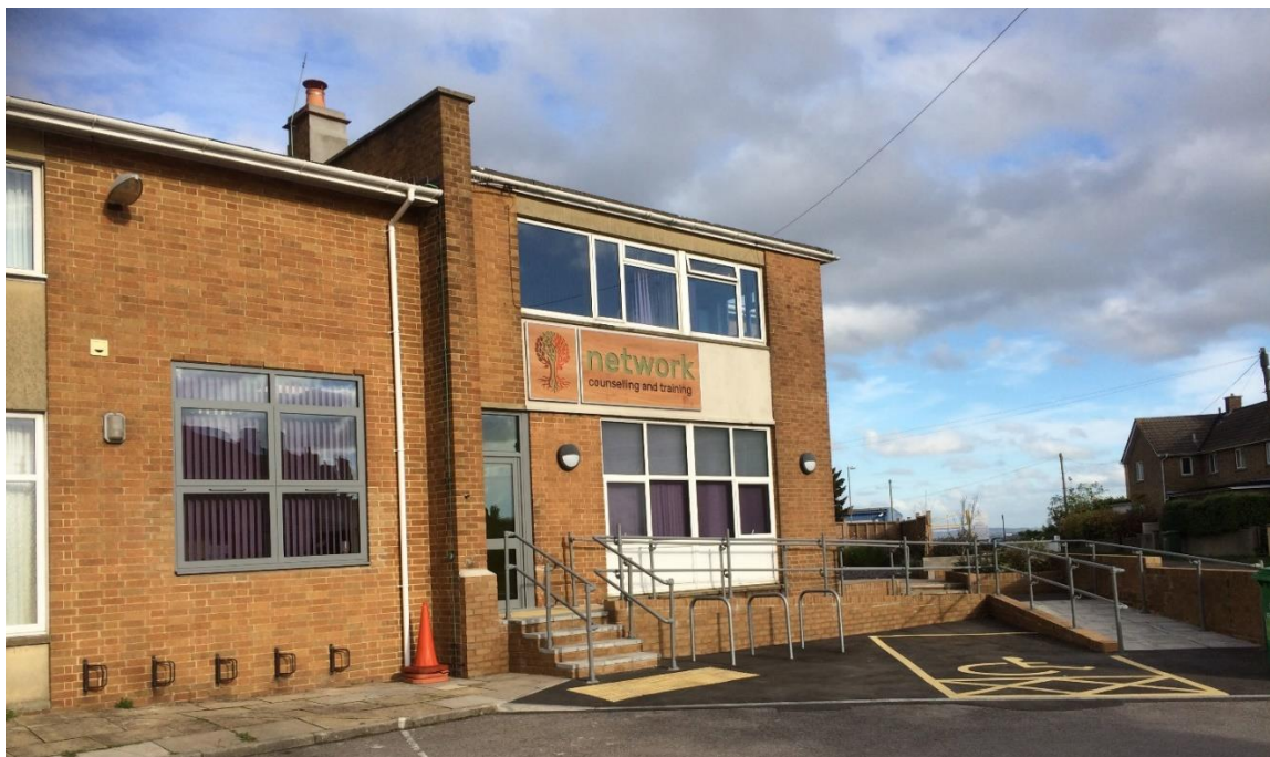
Network at Elm Park, Filton
