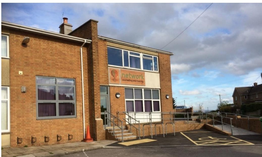
Network at Elm Park, Filton
